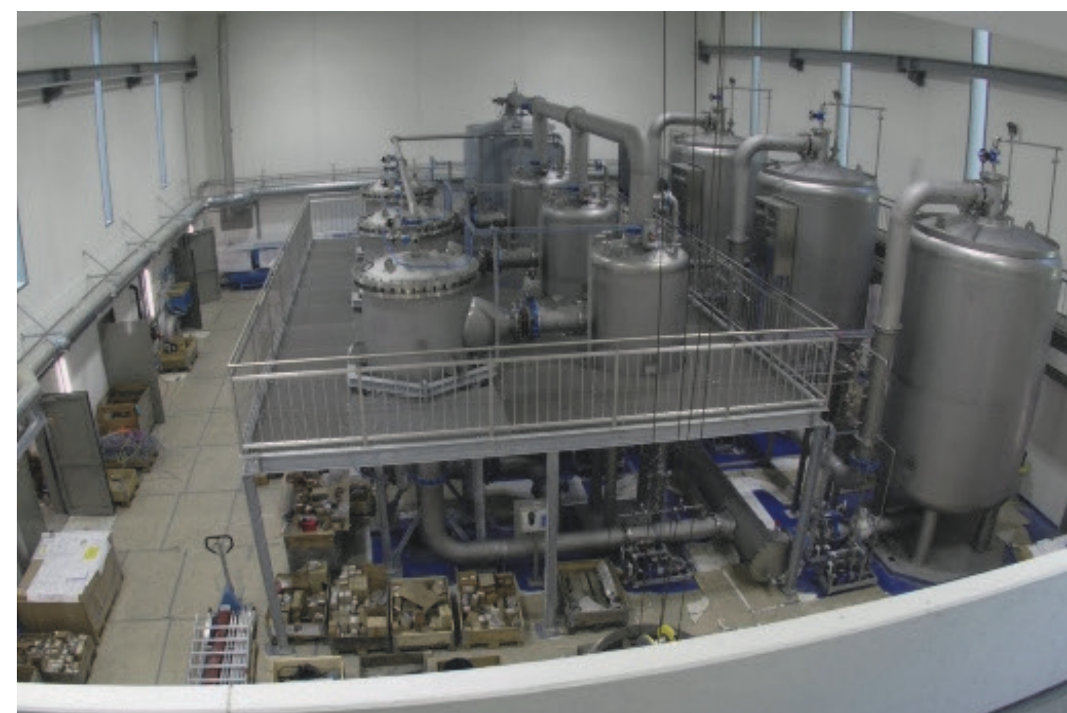
CeraMac® C-37 installation Sonnenberg WTP, ewl energie wasser luzern, Switzerland
